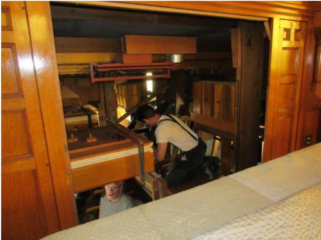
First, the removal of the reservoir
