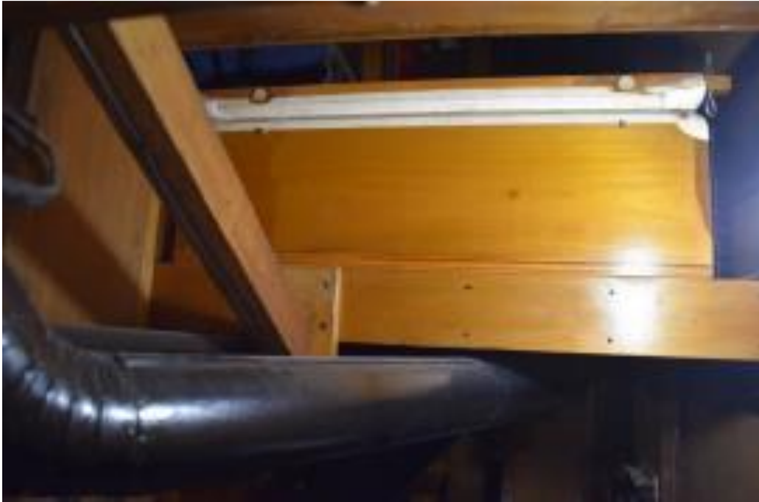
The Choir wind reservoir in place within the organ case.
